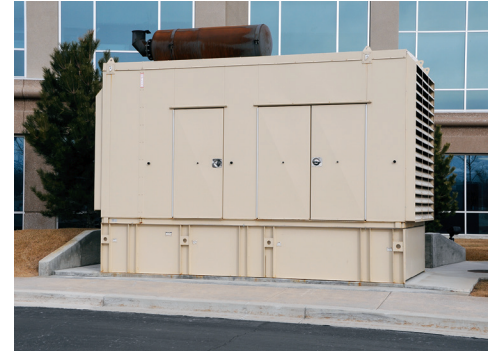
Emergency backup power generator outside of a hospital. Also found serving major office and industrial buildings.
